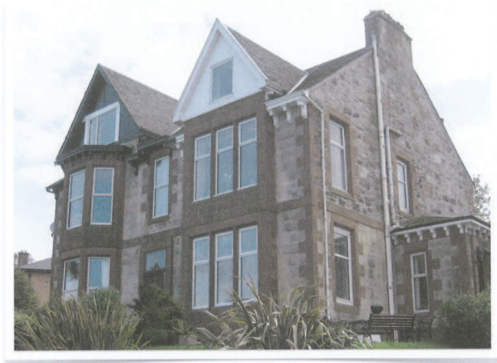
Building 32 - Window Type: UPVC and Various Openings
