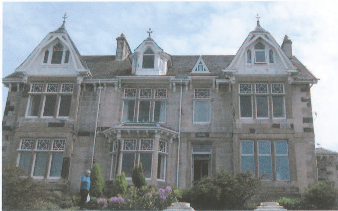
Building 13 - Window Type: Aluminium, Original Installation and Various Openings
