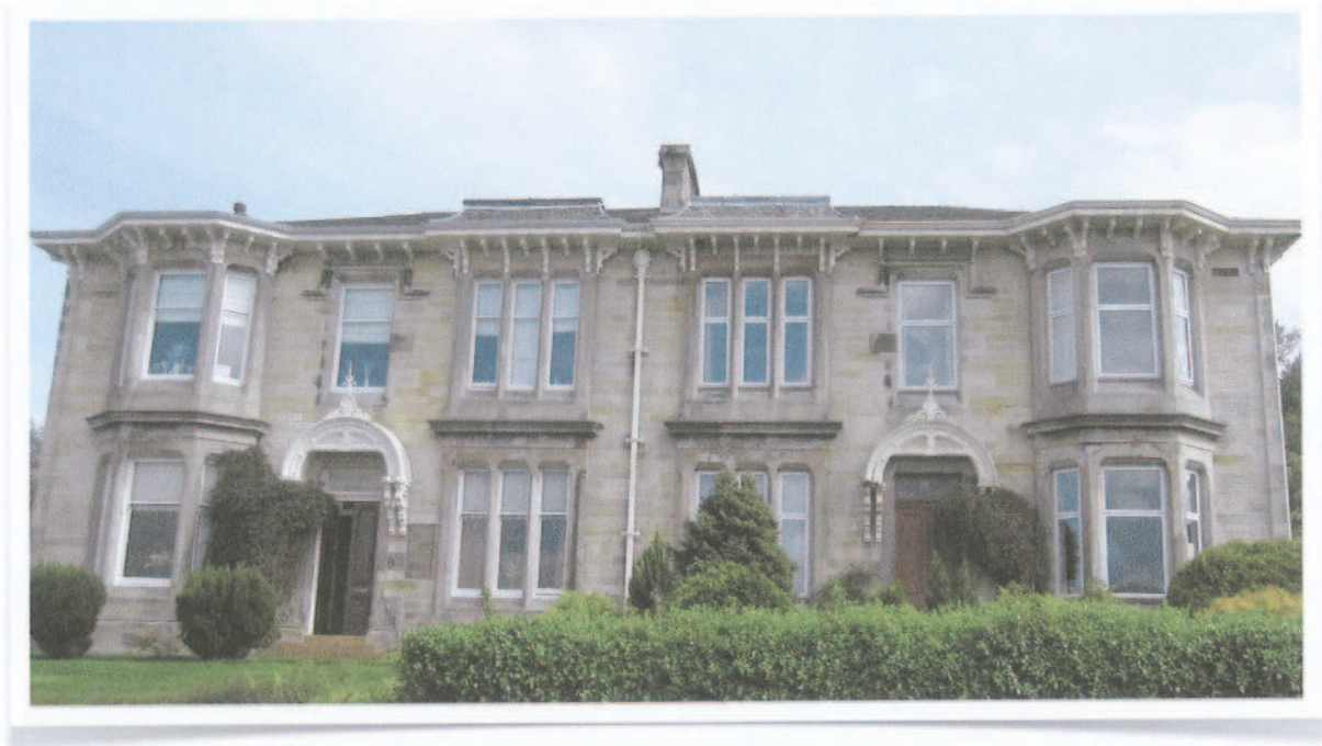
Building 7 - Window Type: UPVC, Aluminium, Original Installation Various Openings
