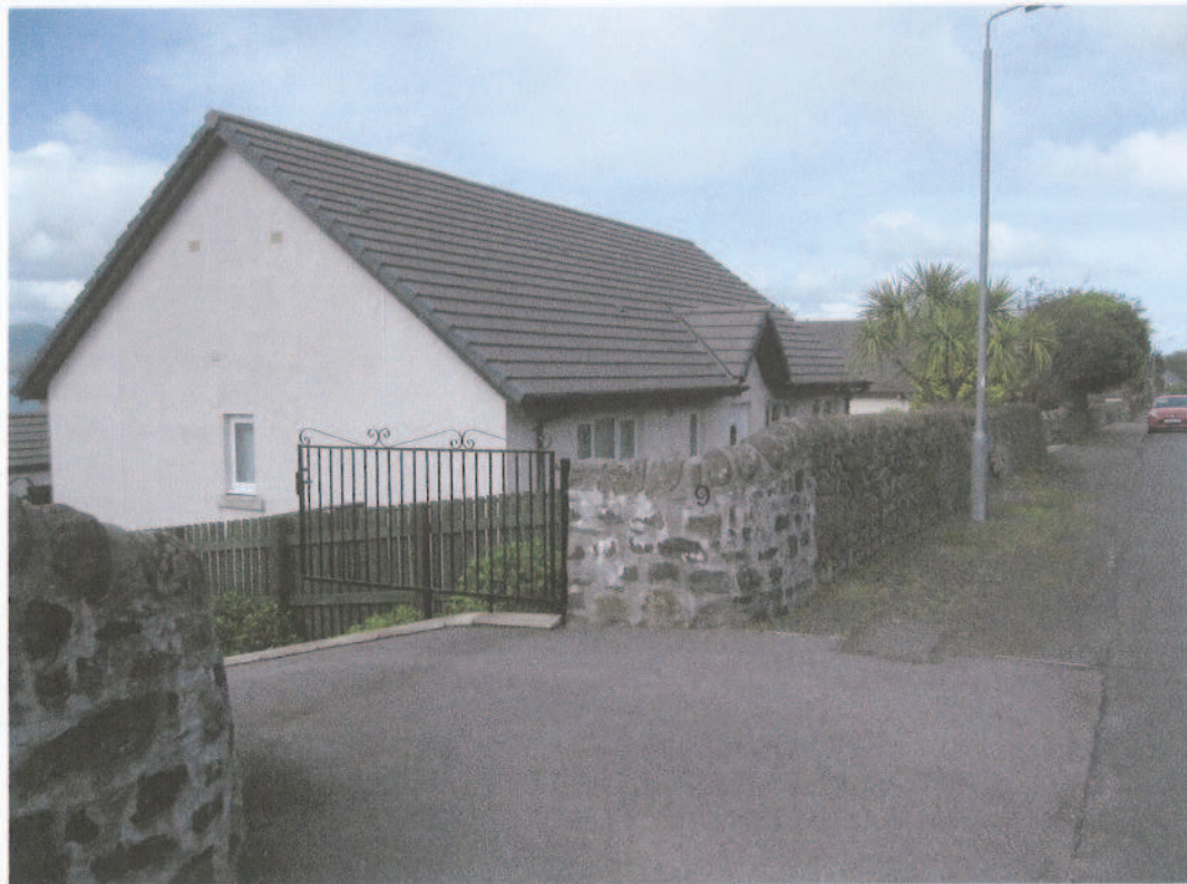
Building 6 - Window Type: UPVC, Various Openings Not Sash & Case
