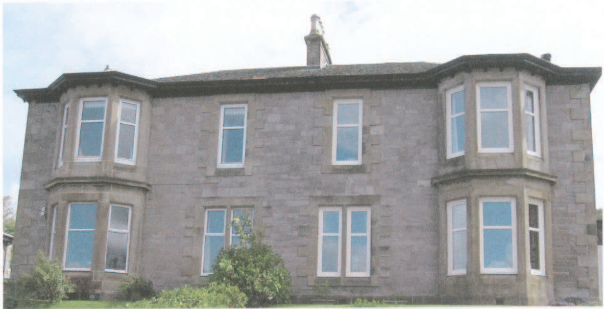
Building 30 - Window Type: Aluminium, UPVC and Various Openings
