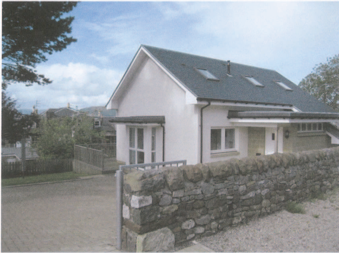
Building 11 - Window Type: UPVC Various Openings
