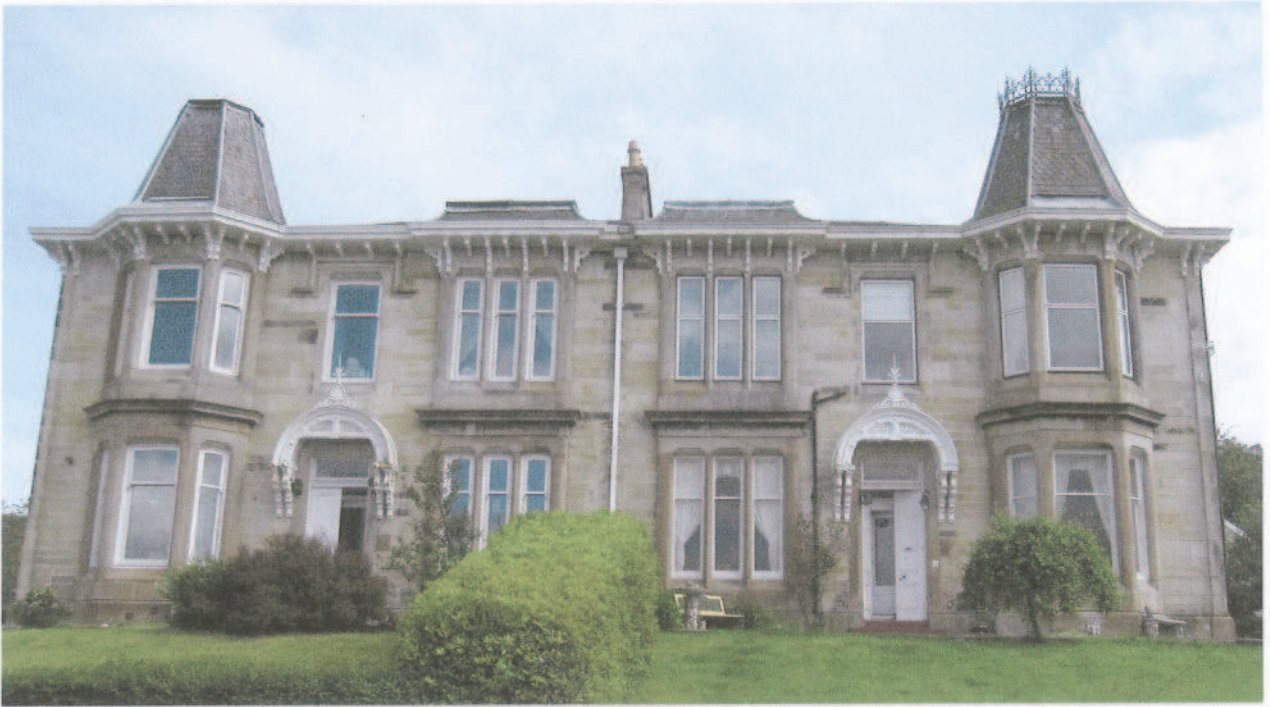
Building 9 - Window Type: Wood Double Swing, Aluminium, Original Installation and Various Openings
